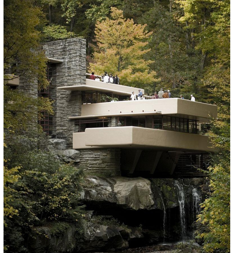
Fallingwater by Frank Lloyd Wright (1937)
